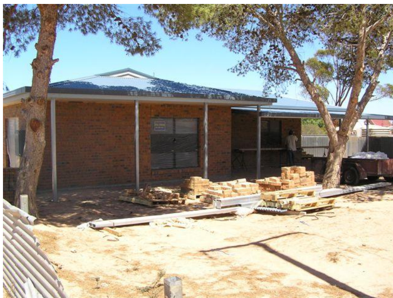
Figure 15: Community house undergoing upgrade, 2007, Koonibba, SA
