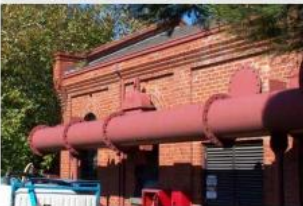
Valve House Existing Valve House building
