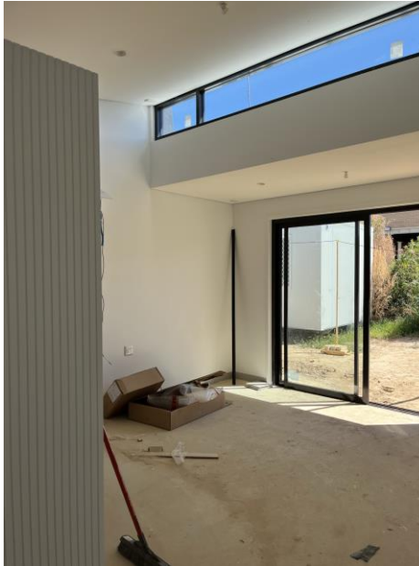
TYPICAL INDEPENDENT UNIT LIVING AREA CONSTRUCTION PROGRESS PHOTO (FEB 2022)
