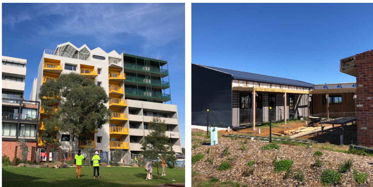
Figure 13: Nightingale Village (left) and The Cape (right) construction sites: January 2022
