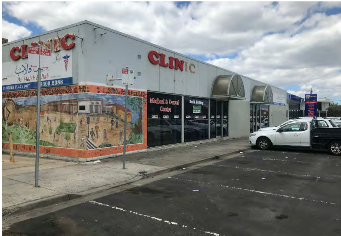
Figure 15: Run-down local amenity nodes are coupled with grade parking
