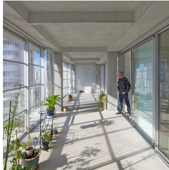
Adaptive Reuse, Bordeaux, France Architect: Lacaton Vassal
