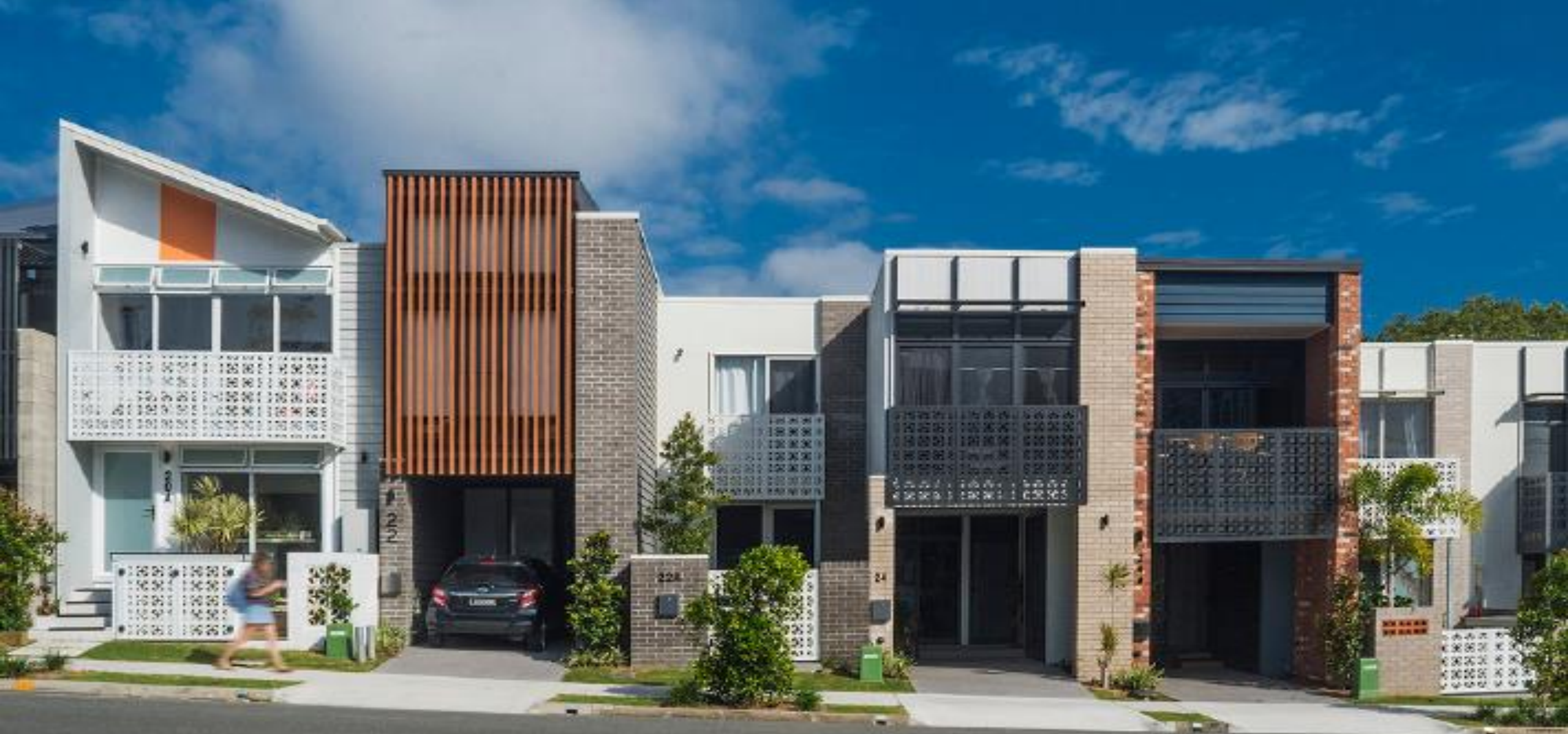
ENVI Micro Urban Village is a multi-award winning micro-lot development in Southport, Queensland, designed by degenhartSHEDD and developed by bubbli(up). This project demonstrates density done well. Photographer Tom Anthony.
