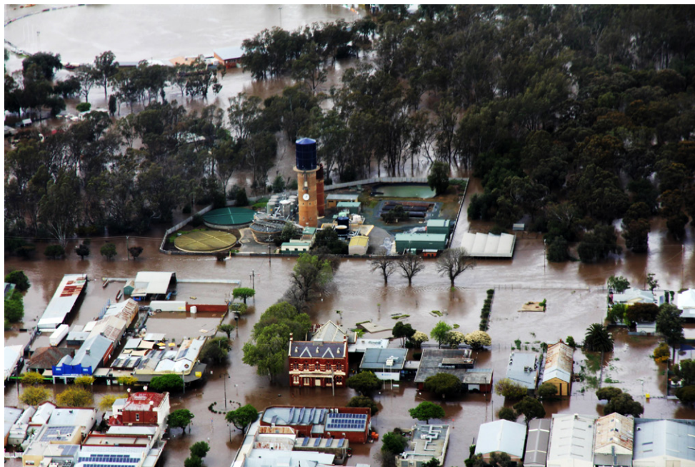
Figure 10: Water treatment plant during the floods, Rochester
