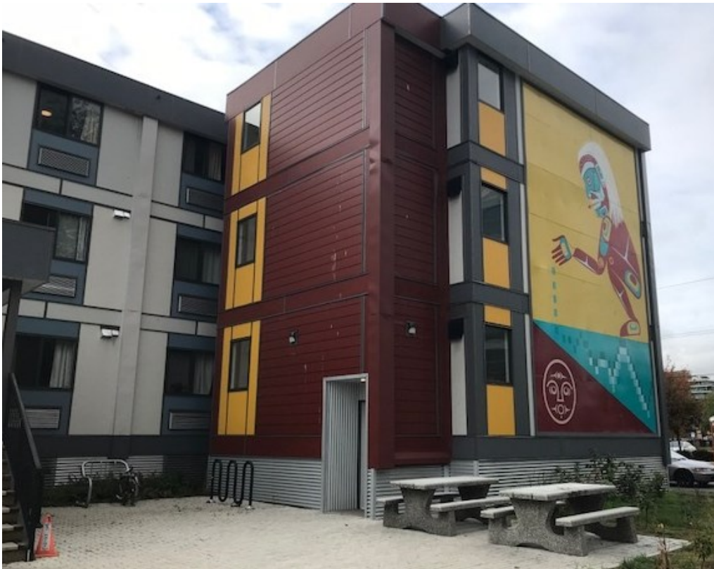
Photo 5: Temporary modular housing at 220 Terminal Avenue
