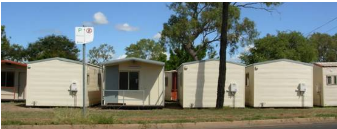
Figure 24: On-site cabins at Moranbah Caravan Park
