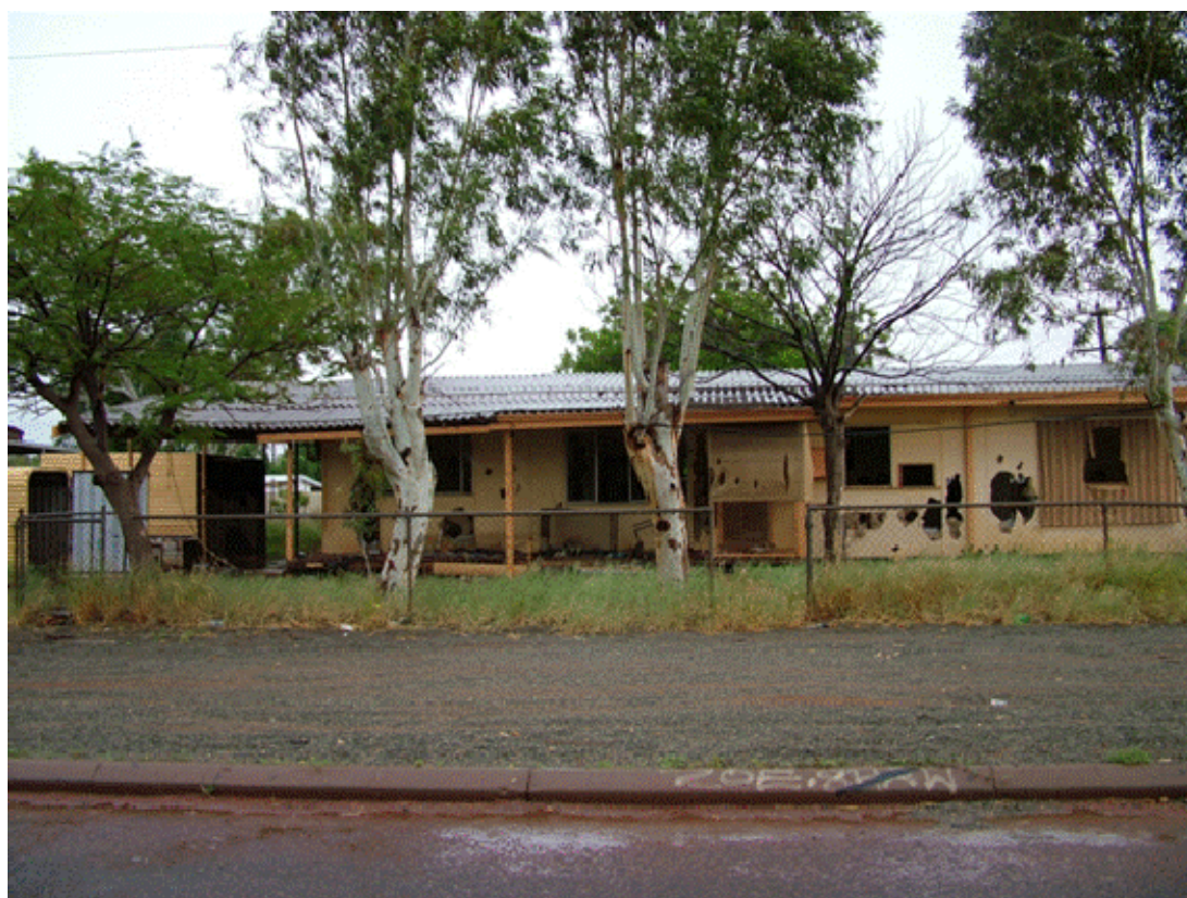
Figure 10: Roebourne house, left vacant and subsequently vandalised
