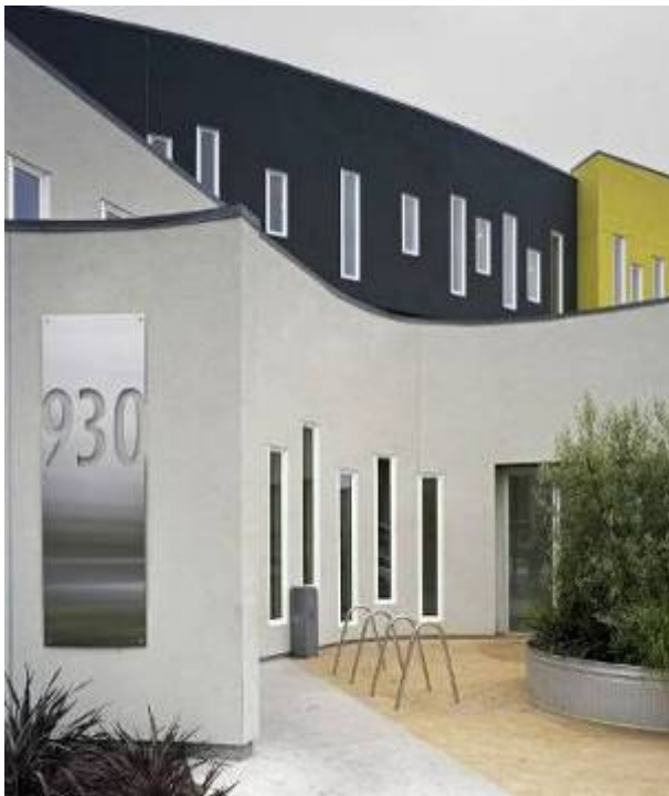
Detail of the community room and apartment entry.
