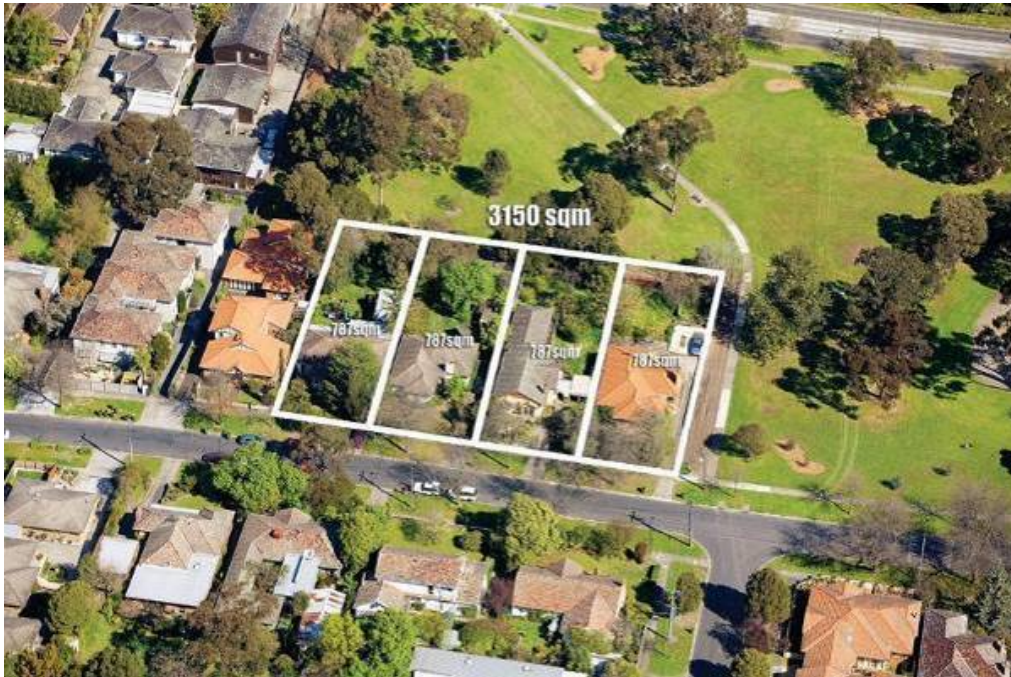
Figure 17: Boisdale Street redevelopment
