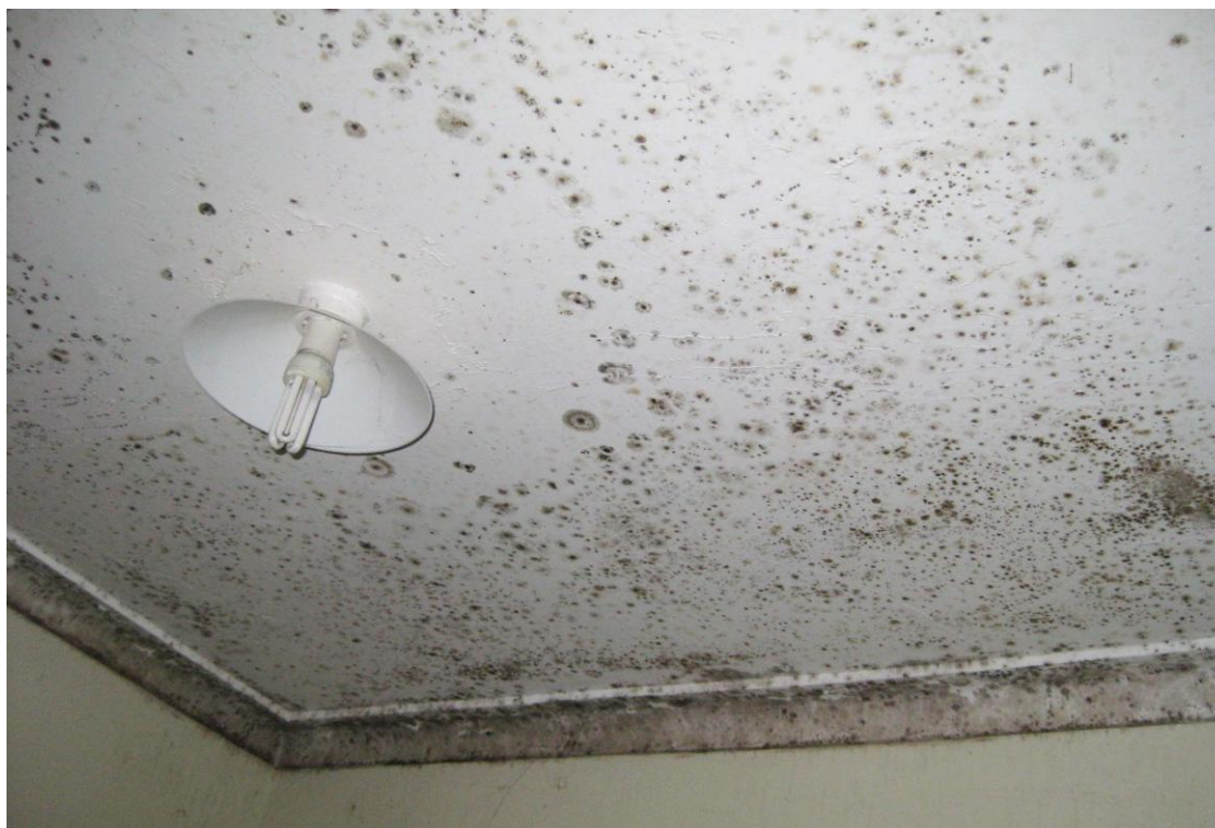
Figure 14: Mould on ceiling in Inala resident's state government house, caused by inadequate ventilation and poor construction
