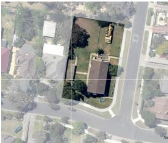
Figure 7: SHI case study—aerial view before
