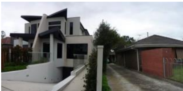
Figure 41: New and old dwelling development
