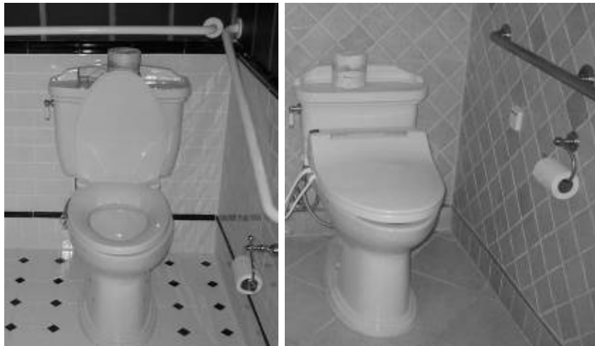
Figure 37: Grab rails in bathrooms
