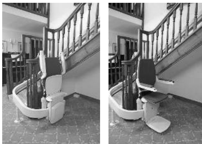
Figure 32: Staircase modified with a stairlift
