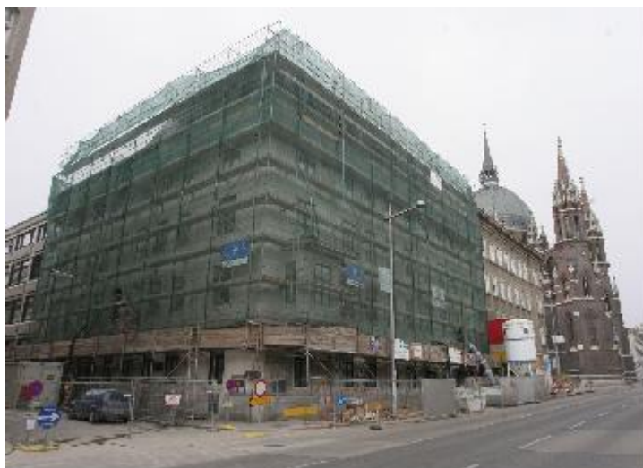
Figure 6: Renovation of older apartments in Vienna (City of Vienna/Ludwig 2009)
