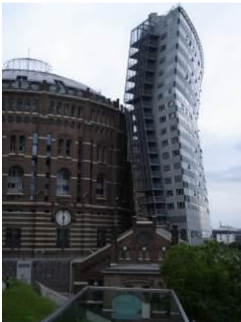
Figure 11: The redevelopment of the Gasometer towers in Vienna, shopping complex with a variety of housing tenures (Lawson 2008) 17
